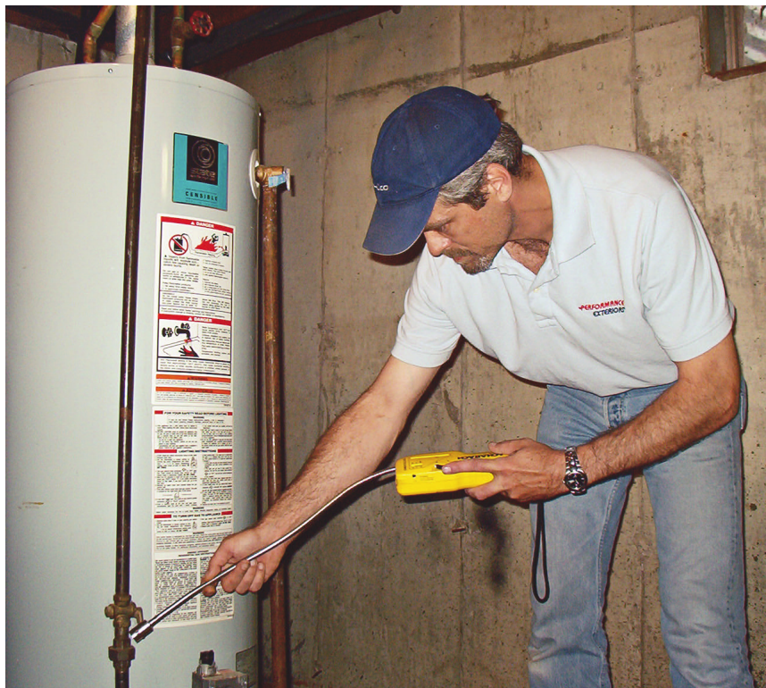
Michael Lotesto tests water heater gas lines for leaks.
